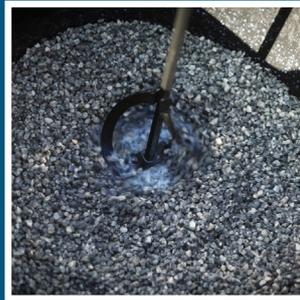
2. Mix EASIHOLD with your stones until they are evenly coated. You can mix using a mixing paddle, or simply by shaking and rotating the stones using a gauging trowel until fully coated throughout.
