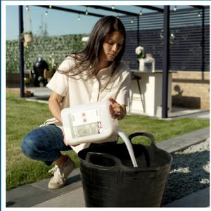
1. Mix EASIHOLD together with your stones in a mixing bucket. Each 5L EASIHOLD mixes 6 x 25kg bags of stone or approximately 1 part of EASIHOLD to 25 parts stones by volume (Jug / Bucket Fulls).
