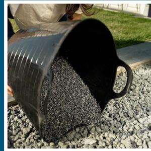
3. Pour out the EASIHOLD mix on to a permeable base. A permeable base is important to allow rainwater to drain through. The overall depth of EASIHOLD treated stones should be 20mm.
